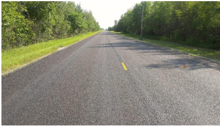
Figure 2 - TH 89 after placement of chip seal
